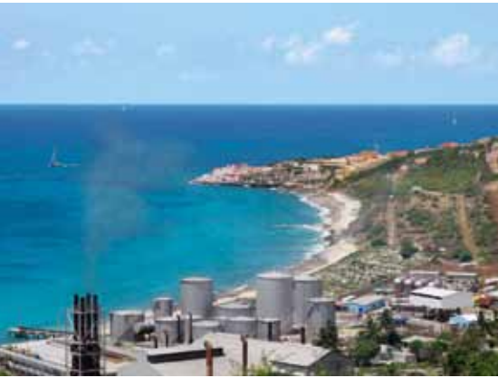
Desalination plants - a less commonly known application area of duplex stainless steel and ESAB consumables.
