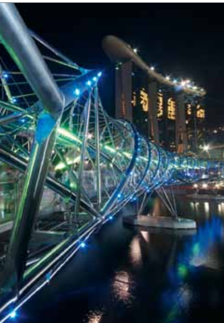
Bridges - a relatively new application area of duplex stainless steel.
