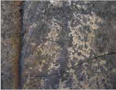
Transverse cracks in a hardfacing layer.
